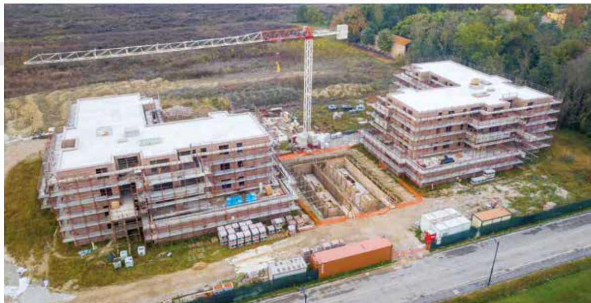
Intervento Social Housing 40 alloggi a Molinella (BO) - 2020
